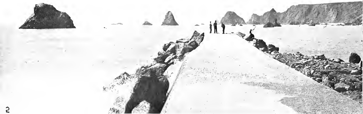
Views of rock and concrete jetty at Jenner that is keeping open Russian River channel to ocean
